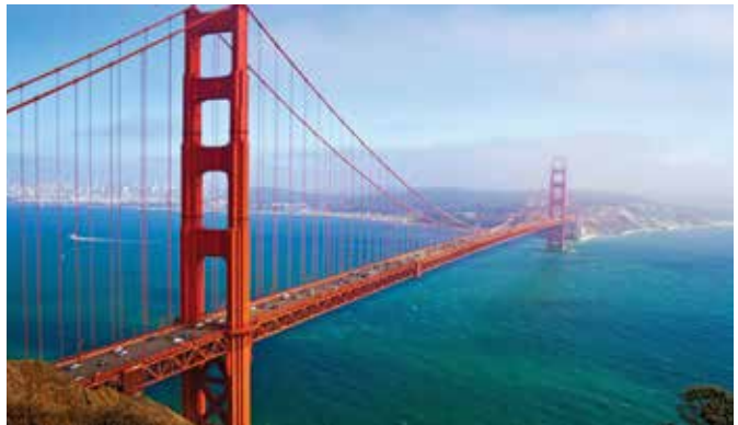
Golden Gate Bridge
